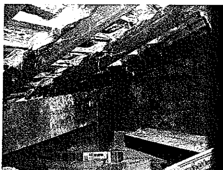
Figure 2: Roof void at rear
