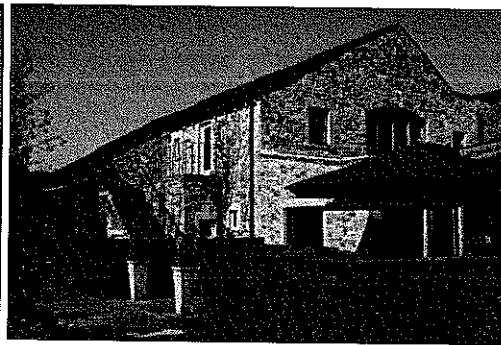
Barn from south east
