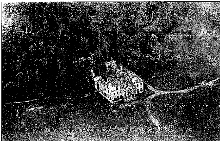
Woodfold Hall before restoration
