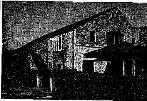
Barn from south east
