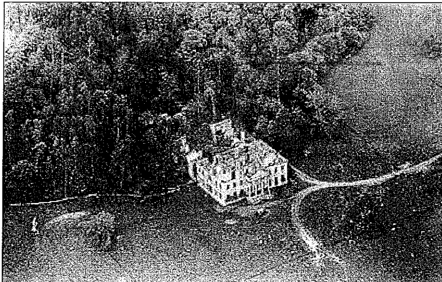
Woodfold Hall before restoration
