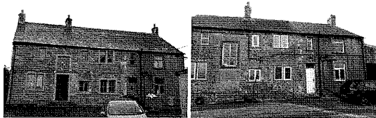
Farmhouse showing the C19th extension to the rhs, (brickwork with roughcast render). Facade recently repointed and entrance door reinstated.
