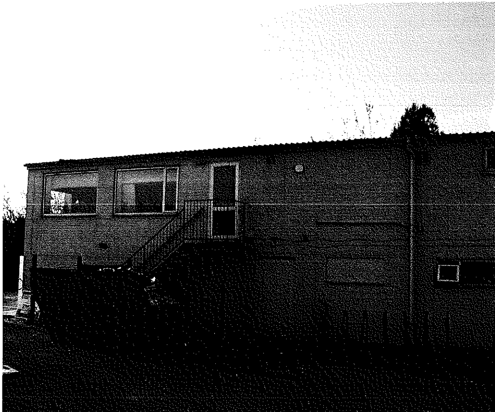
Part North East Elevation on which it is proposed to construct the open viewing terrace.
