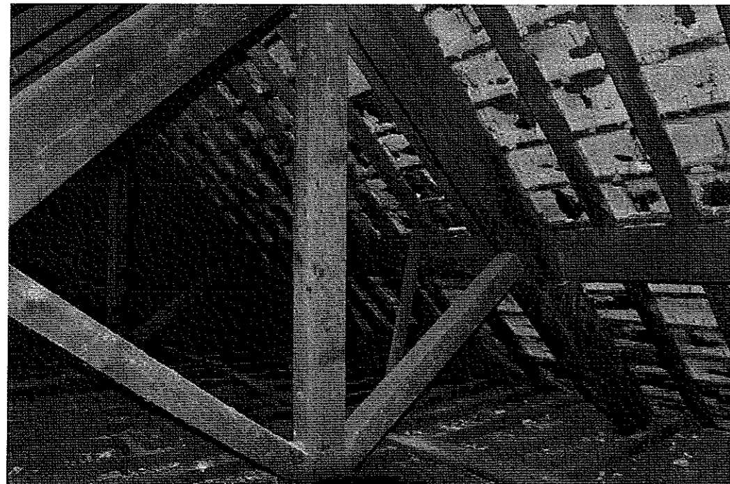
View of east roofspace. April 2010.
