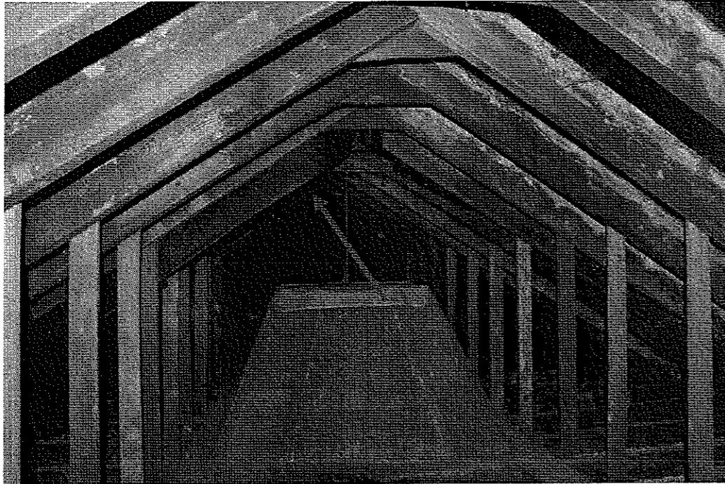
View of west roofspace – bat roost marked with red arrow. April 2010
