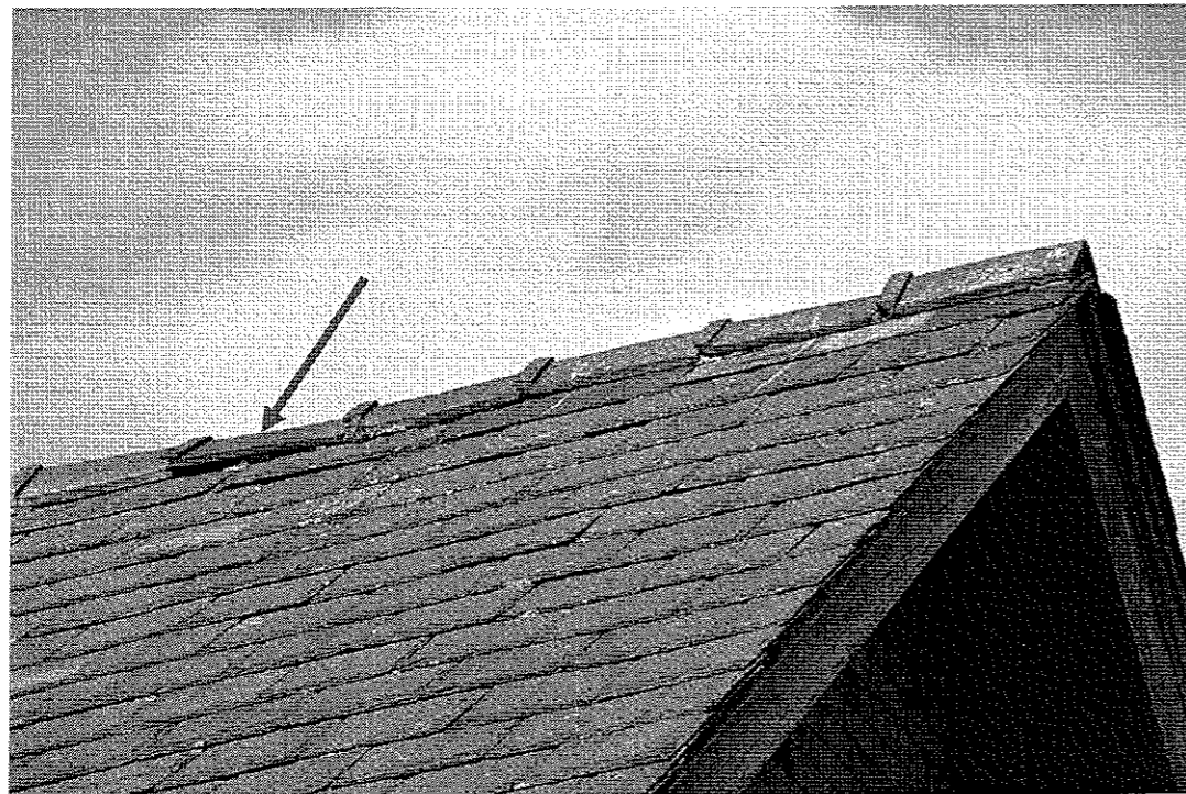
Ridge tile emergence point above south elevation. May 2010.
