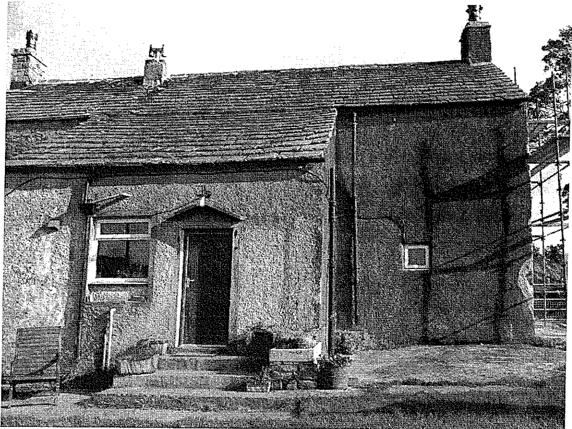
Figure 2: Photograph of existing rear elevation
