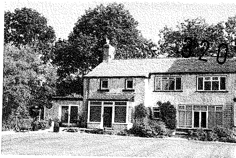
Pl. 13 Photograph showing part of the rear/ north west elevation of Chorley House, taken from the garden, and showing some of the mature trees.
