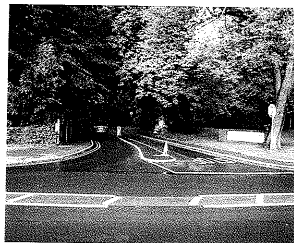
Photo 3 – Existing road junction
