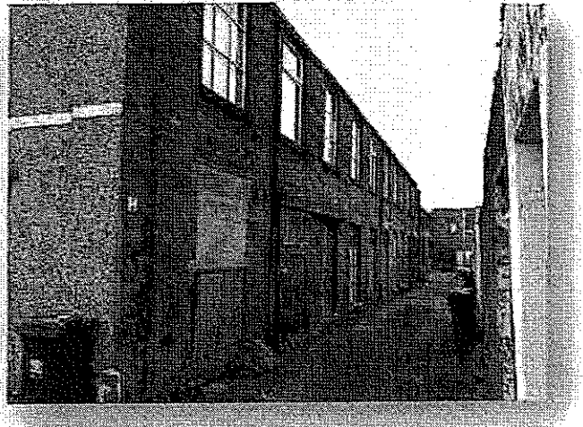
Figure 2 West Elevation down side alley
