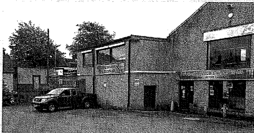
Figure 5 Heavily rendered elevations and ill-conceived signage
