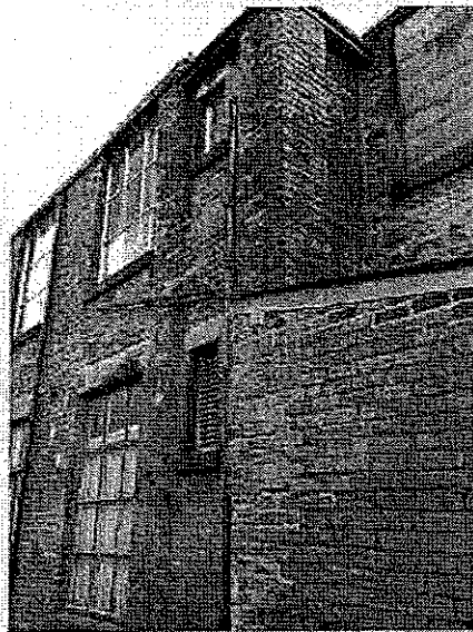
Figure 3 West Elevation down side alley
