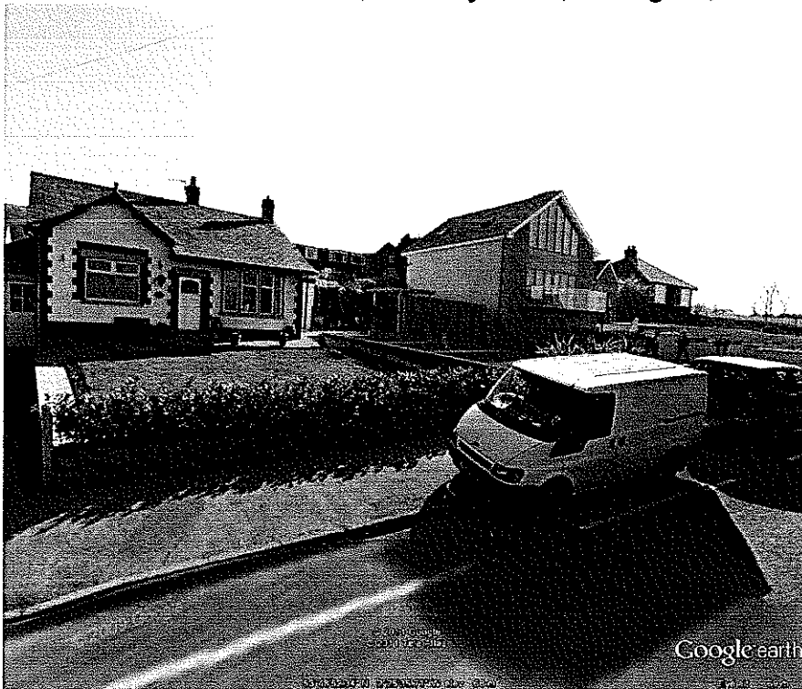
Image 8: Image showing the intensity of the dwelling on the Street scene at Strathaven, Whalley Road, Billington, BB7 9LG
