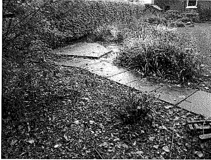
Photograph showing the paths and concrete bases
