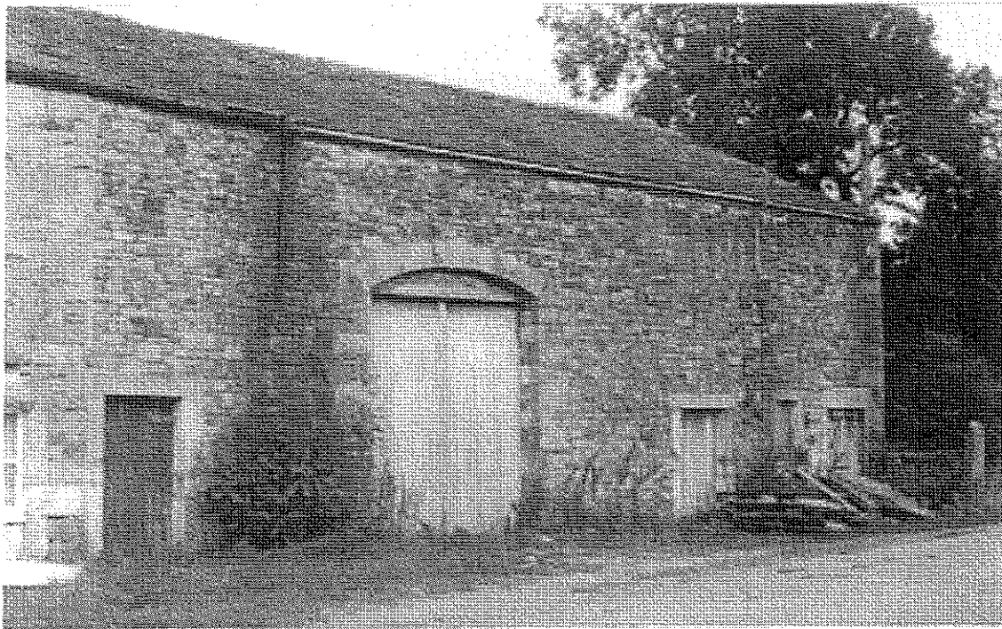
Plate 6 Front elevation of Barn 2
