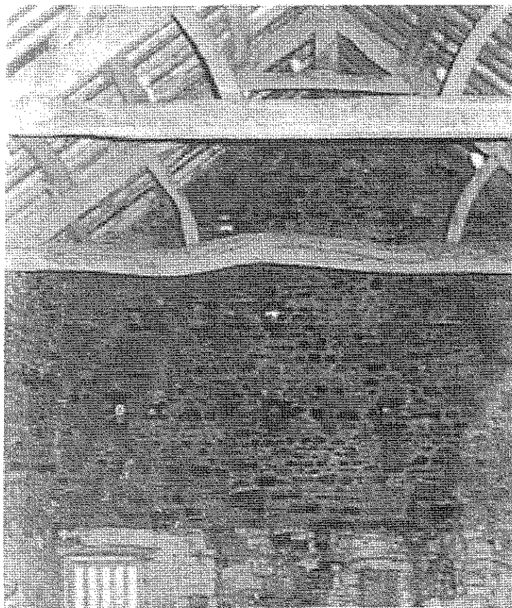
Plate 9 The southern roof trusses of the Old Barn
