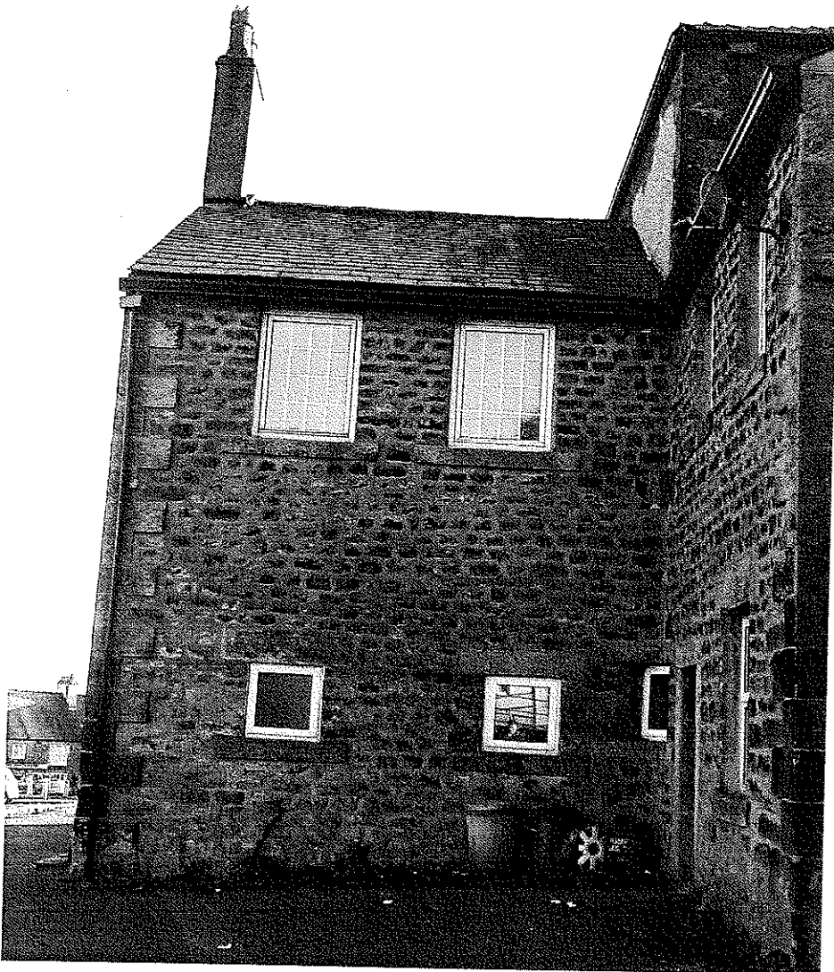
Photograph 32 – Right Side Elevation
