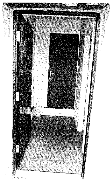
Photograph 1 – View from main entrance door looking into entrance corridor / lobby
