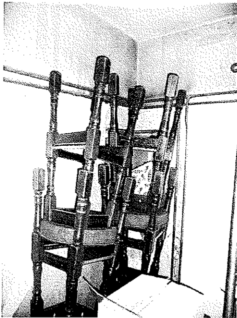
Photograph 21 – Junction of internal wall to meeting room and external wall to left side elevation where window is situated
