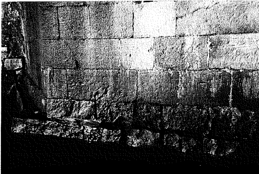
P13 OPEN JOINTS IN BOTTOM COURSE WITH HAIRLINE CRACKING OF BLOCK 29677/6/11
