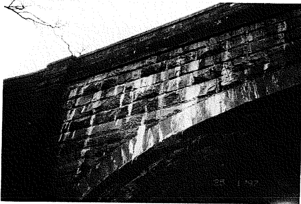
P29 WATER STAINING OF NORTH MIDDLE ELEVATION SPANDRELS
