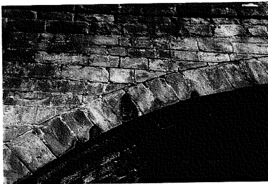
P23 WATER STAINING AND MORTAR LOSS IN SOUTH WEST ELEVATION
