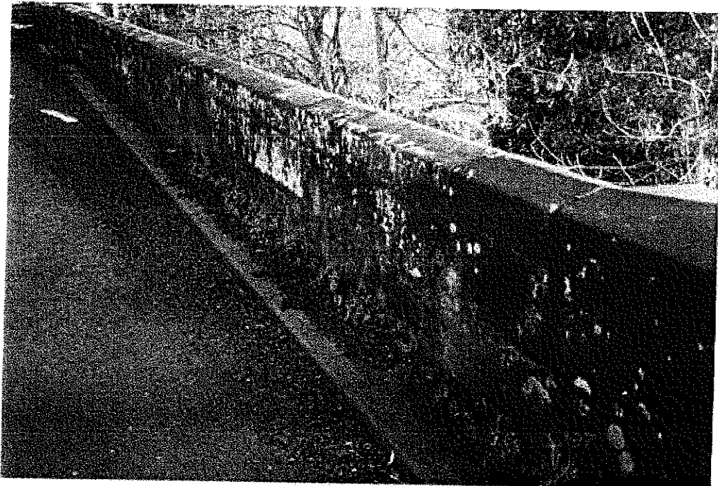
P32 VEGETATION GROWTH ON ROADSIDE OF SOUTH EAST WING WALL
