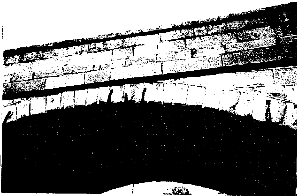
29. Water seepage at crown and leached deposits
