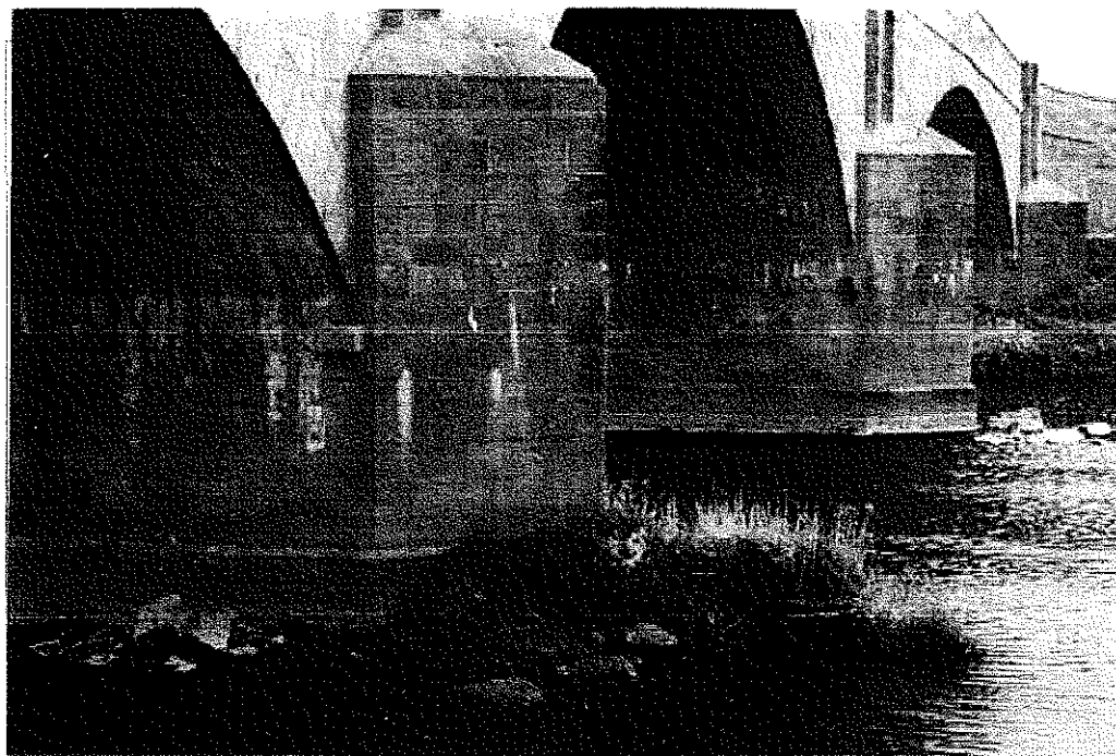
P2, East and West Piers - Areas of lichen growth and leaching. Vegetation at bottom of West Pier.
