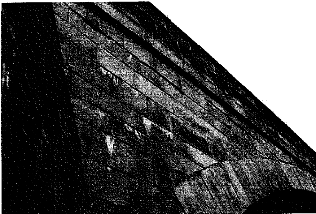
P16. Spandrel, span 1, north - Areas of mortar loss, cracked mortar, leaching and lichen growth. Small horizontal displacement of masonry blocks.
