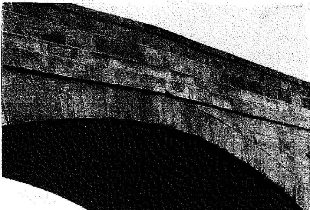
P15. Arch Ring, span 1, north - Loss of mortar, cracked mortar, leaching and areas of lichen growth.
