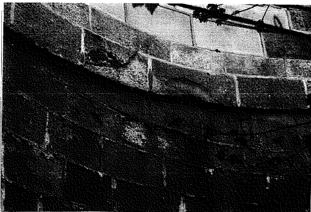
P6. South West Wingwall - Areas of mortar loss especially around stringer.
