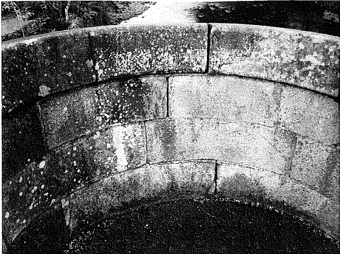
Loss of mortar in parapet joints
