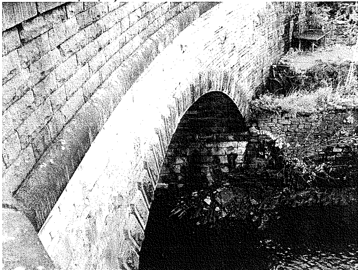
Loss of mortar in parapet joints
