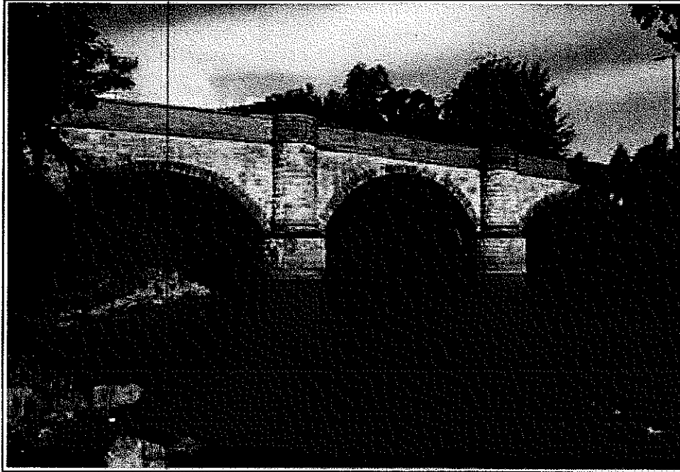
Multiple segmental arch with variable soffit profiles to upstream extension
