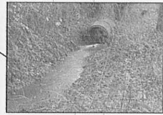
PHOTO 9: Large diameter culvert place in stream.
