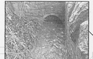
PHOTO 8: Ditch exiting culvert.
