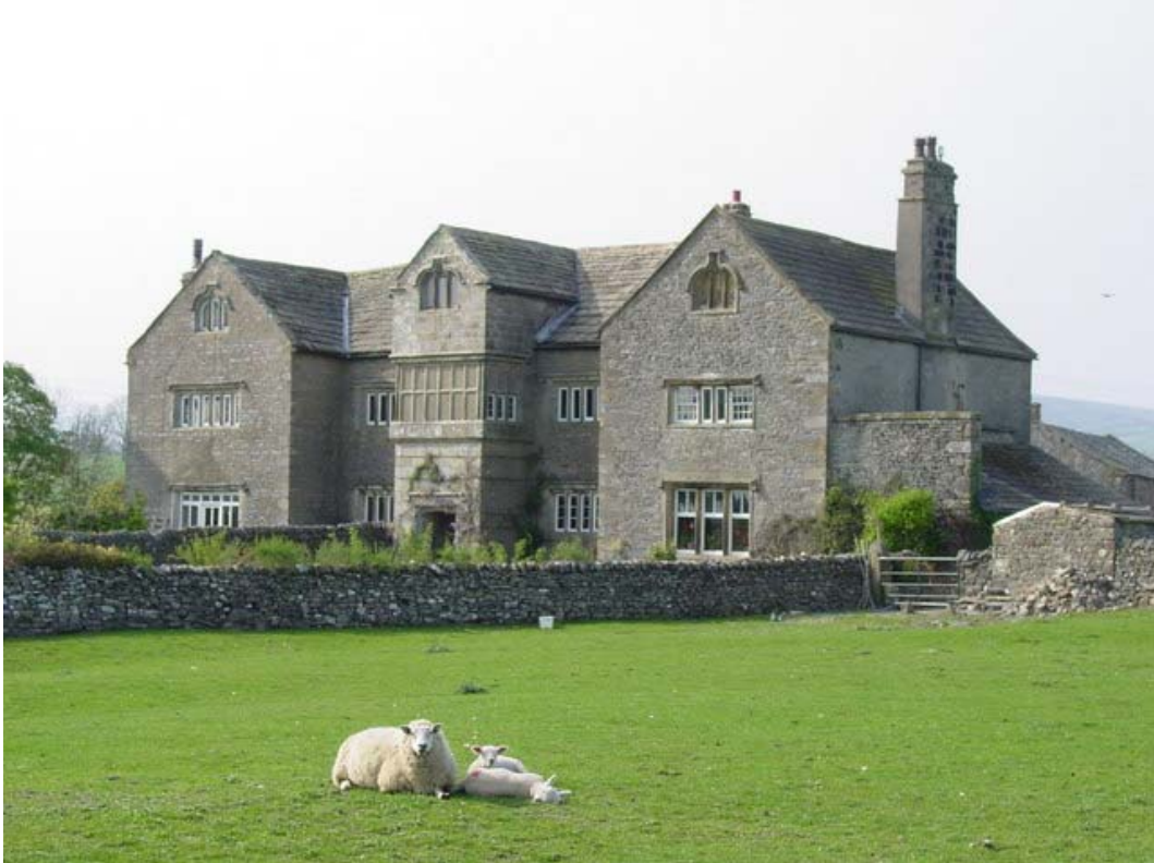
Photo G – Hammerton Hall, Slaidburn
