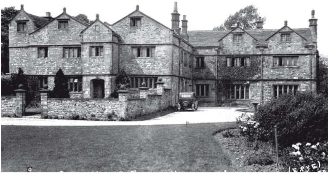
Photo E – Stirk House, Gisburn
