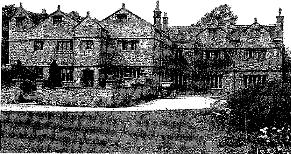
Photo E – Stirk House, Gisburn
