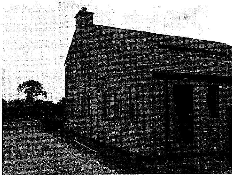
PL 1. Existing South Facing Gable
