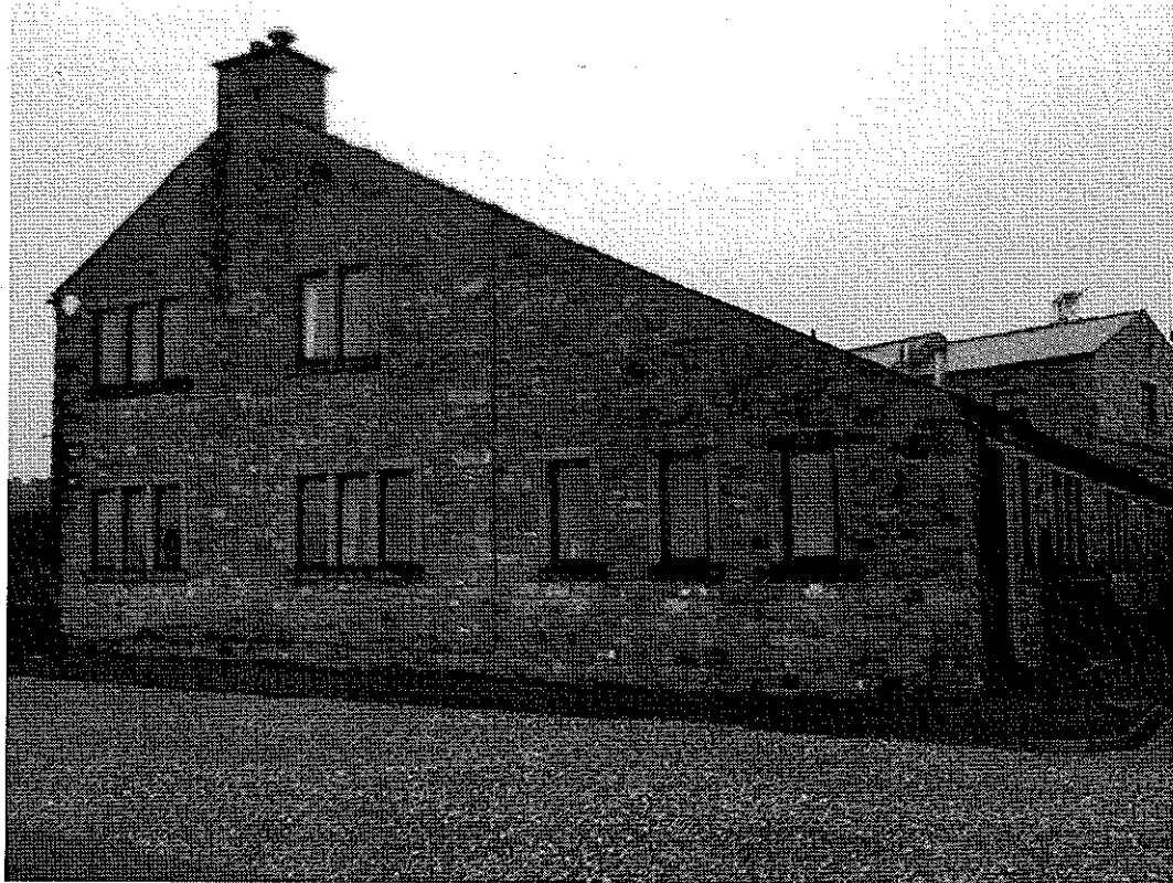
Figure 3: Large uniform windows to ground and first floor of south elevation
