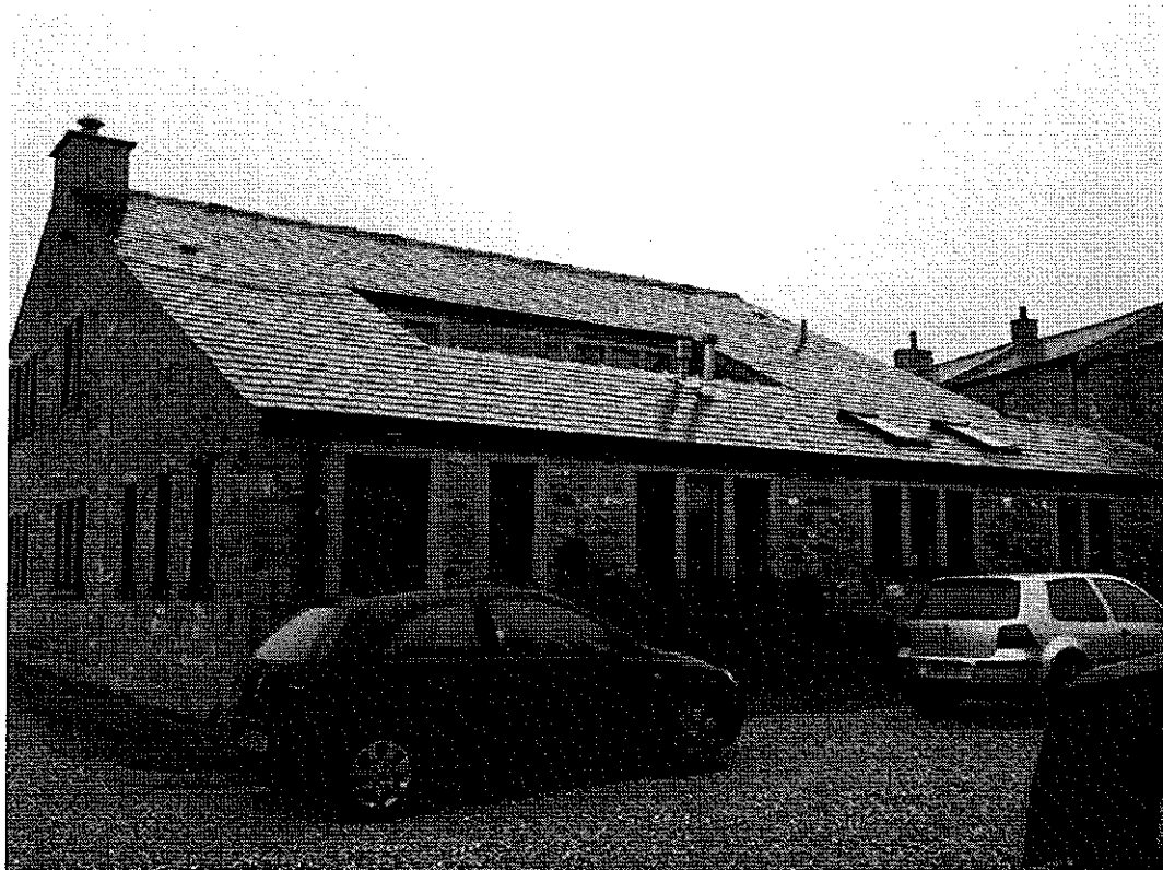
Figure 2: Photograph of east elevation showing gable on projection roof, large domestic windows, inset windows to first floor and roof lights
