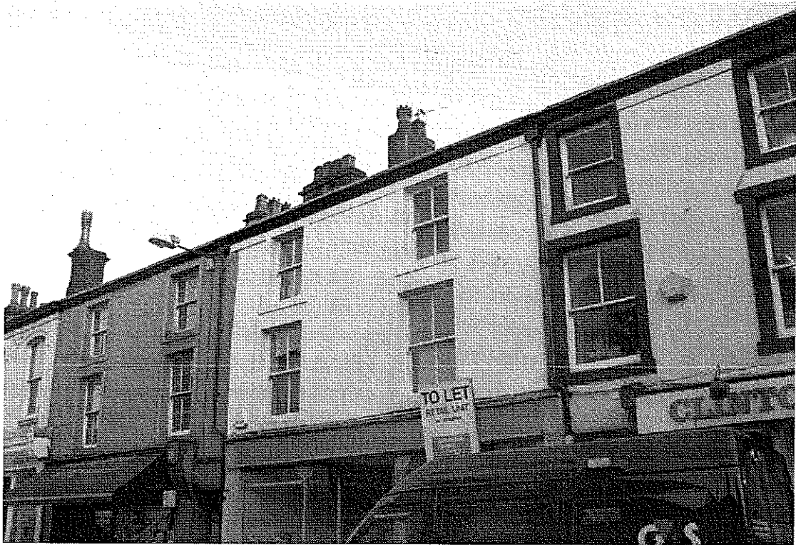
1. Front elevation showing 1 st and 2 nd floor windows
