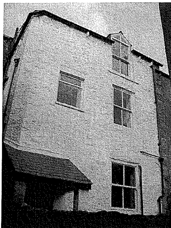
3. Rear elevation of the building
