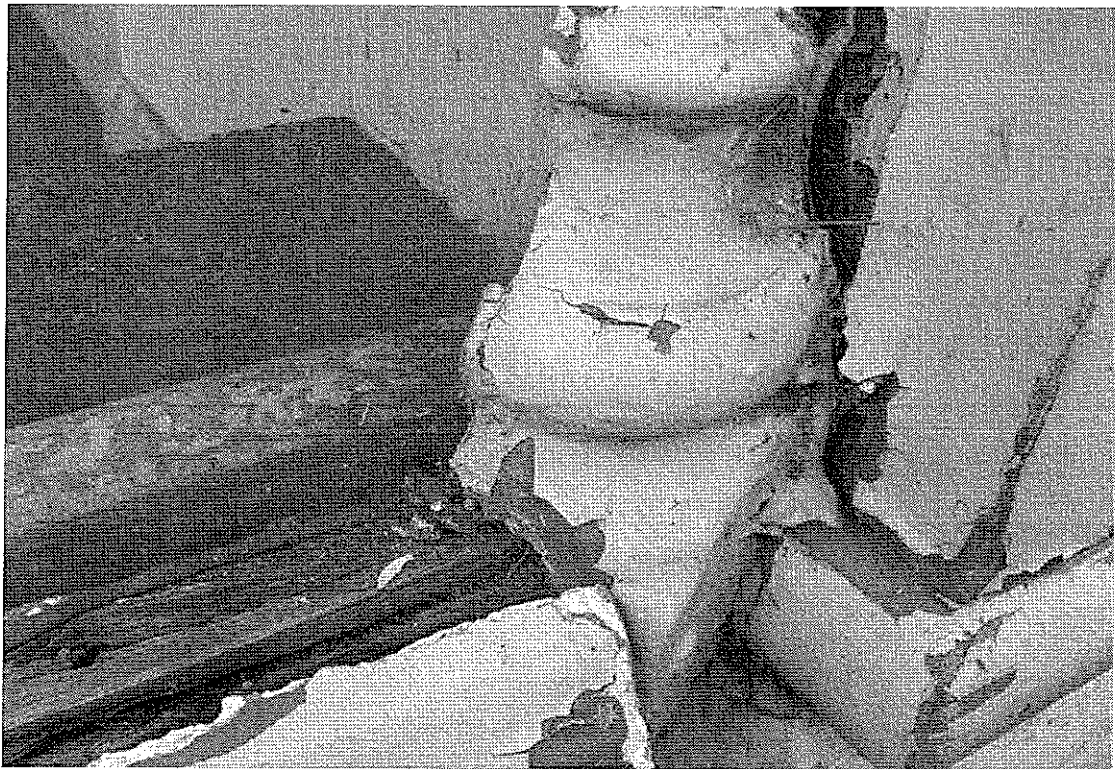
2. Condition of the existing pilaster and mullion detail
