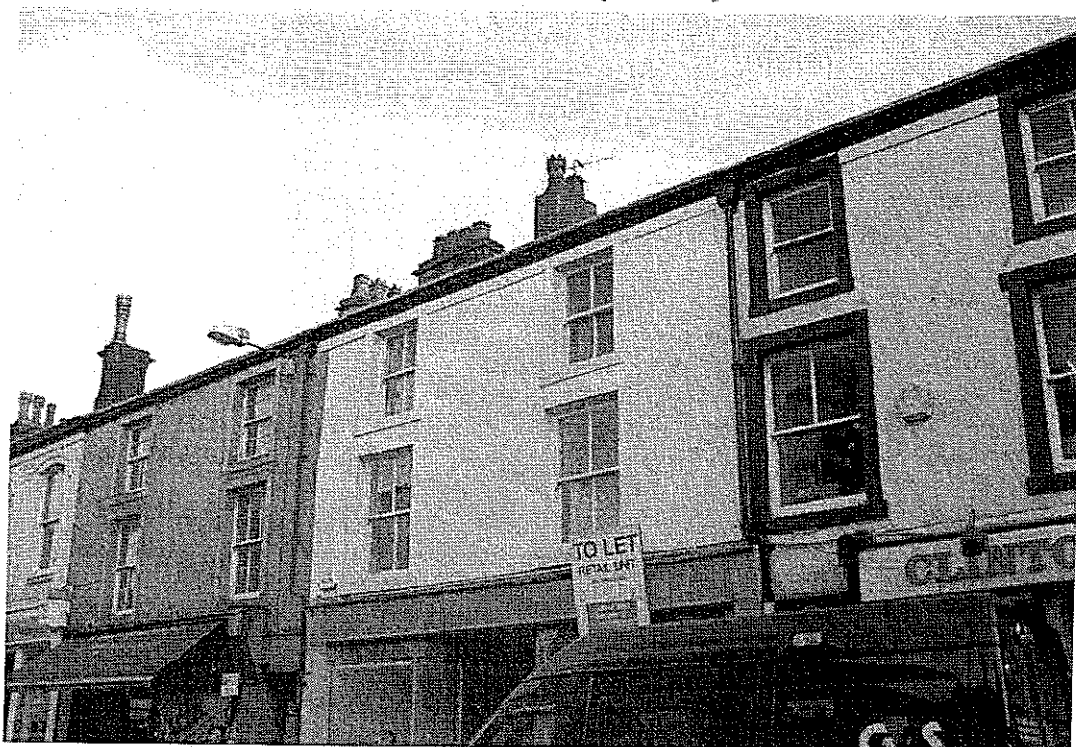
1. Front elevation showing 1 st and 2 nd floor windows
