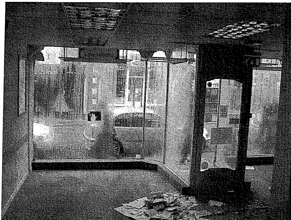
5. Internal view of front of house area
