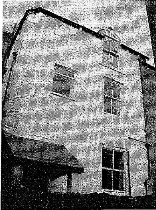
3. Rear elevation of the building
