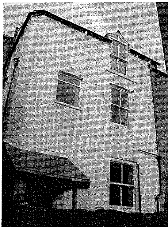
3. Rear elevation of the building
