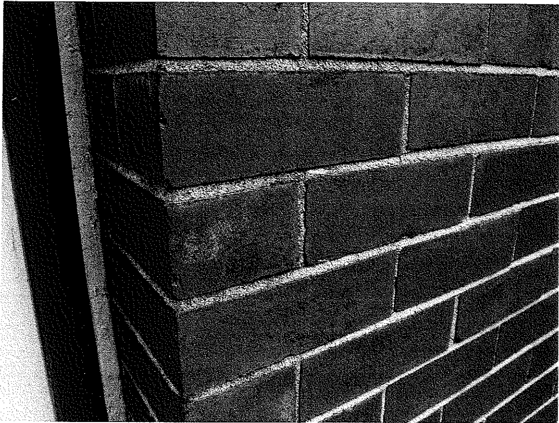
PI. 2 Photograph which shows the sample panel of the brick that would be used to build the external walls of the garage, garden room extension and extended section of the north east wall.
