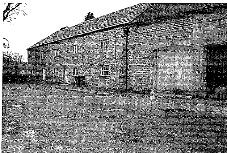
Photograph 2 The north elevation of Browsholme Cotes, with the Listed barn to the right.
