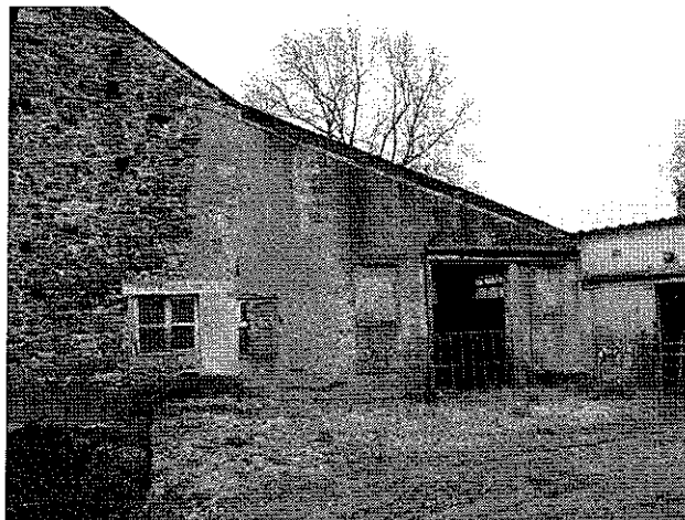
North elevation of lean to
