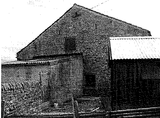
Lean-to on north east gable to be demolished
