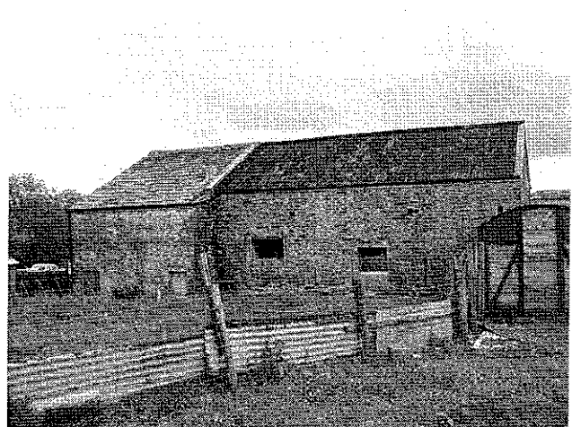
Rear elevation with blocked opening at first floor
