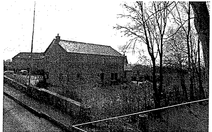
Fig 23. Dilworth Court residential development.
