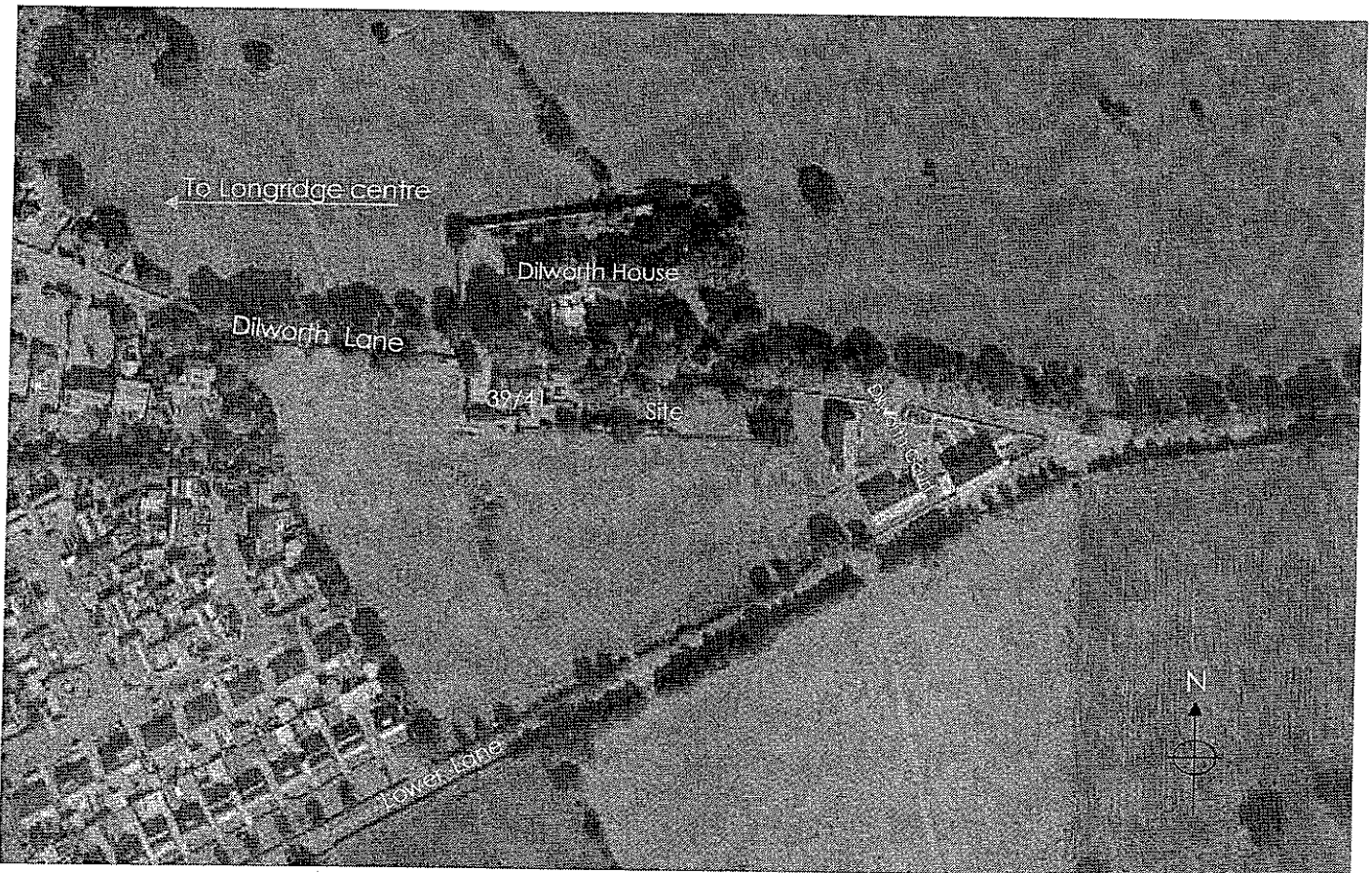
Fig 1. 39+41 Dilworth lane. Aerial view of site.
