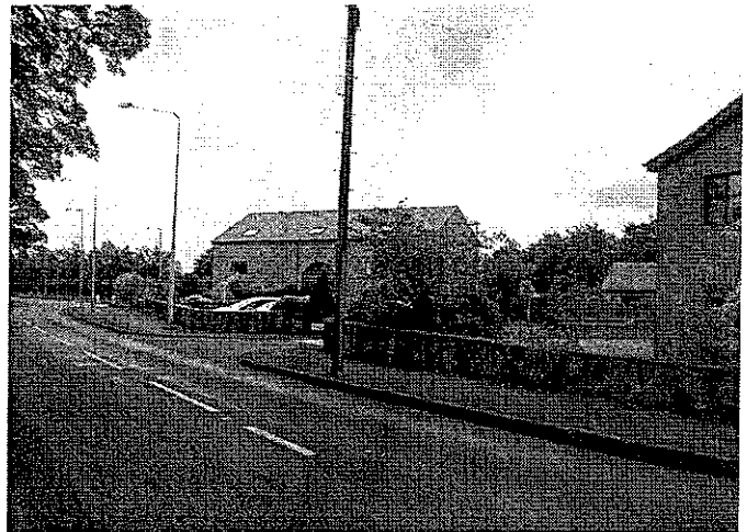
Fig 7. Dilworth Court residential properties
