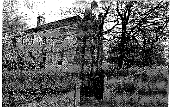
Fig 32. Dilworth House West elevation
