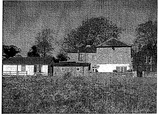
Fig 5. South elevation 39 (left) & 41 Dilworth Lane
