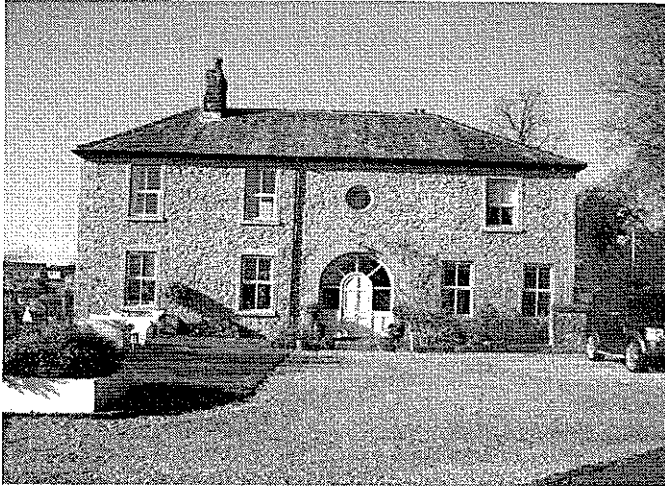
Fig 4 East elevation Gardeners Cottage
