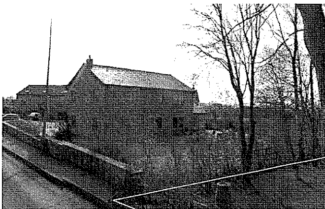
Fig 23 Dilworth Court residential development.
