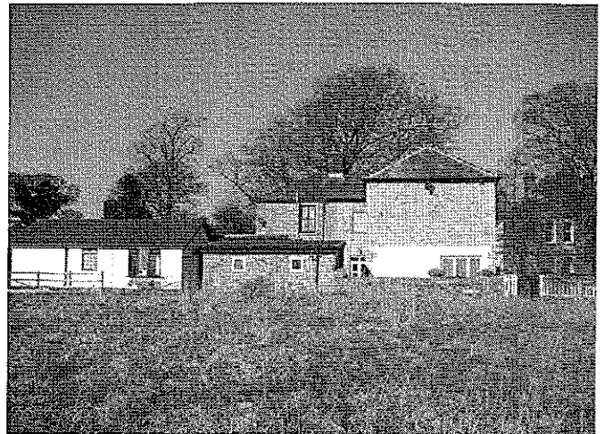
Fig 5 South elevation 39 (left) & 41 Dilworth Lane
