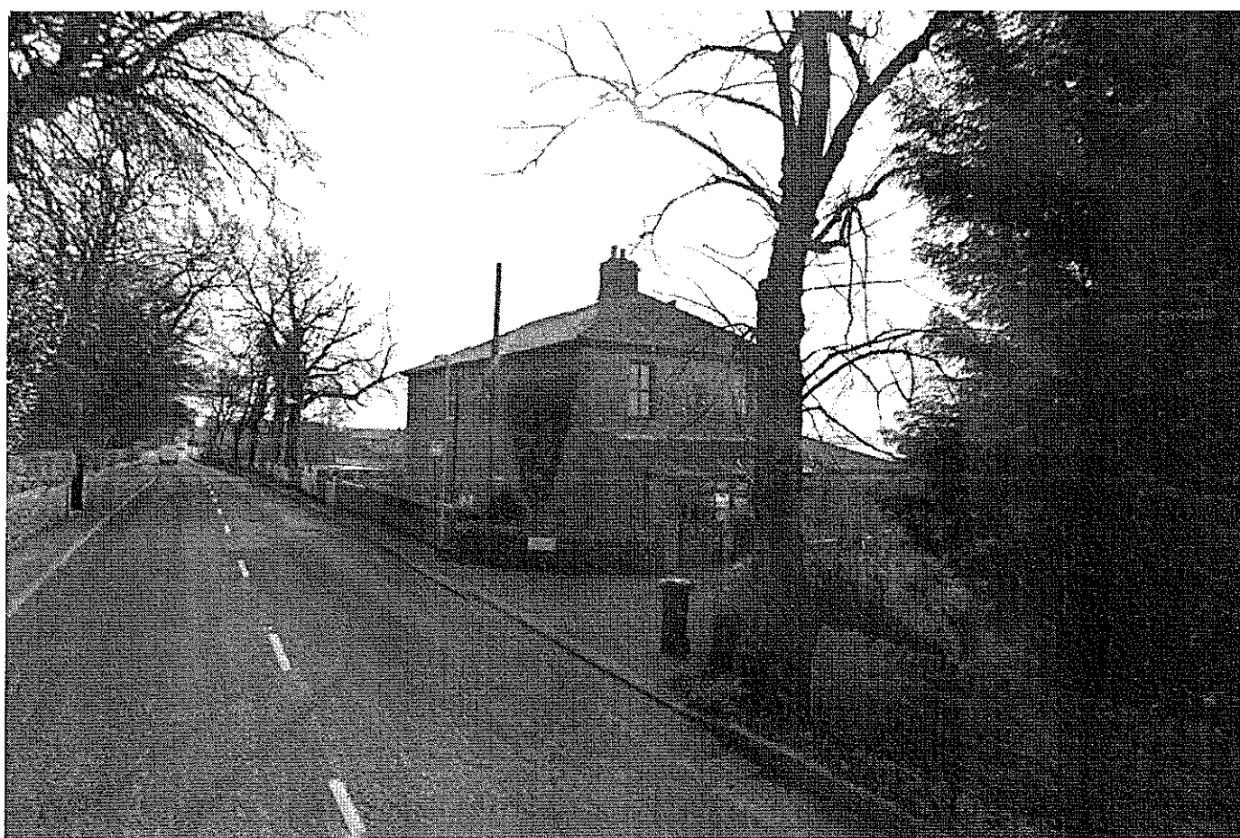
Fig. 35 Same elevation, as seen today depicts the large conservatory addition.
