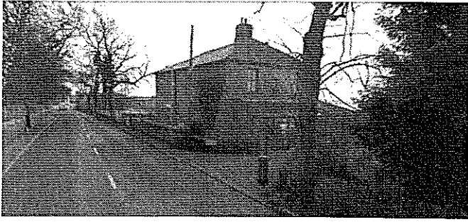
Fig 2 View from Dilworth Lane towards 39 Dilworth Lane
