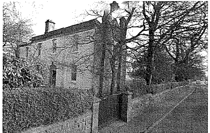
Fig 32 Dilworth House West elevation
