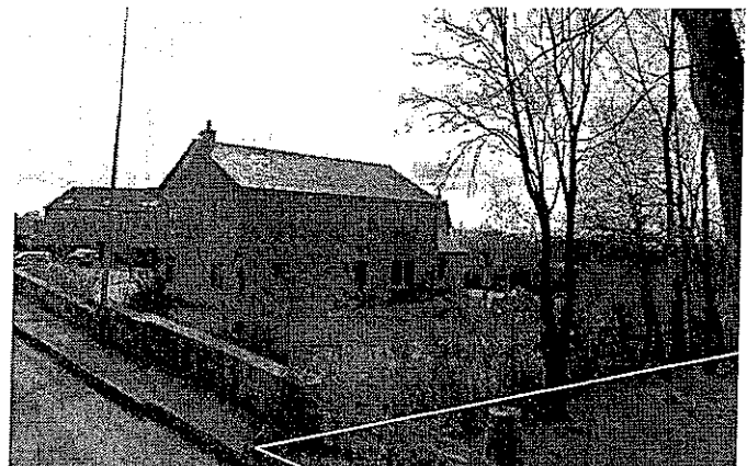
Fig 23. Dilworth Court residential development.
