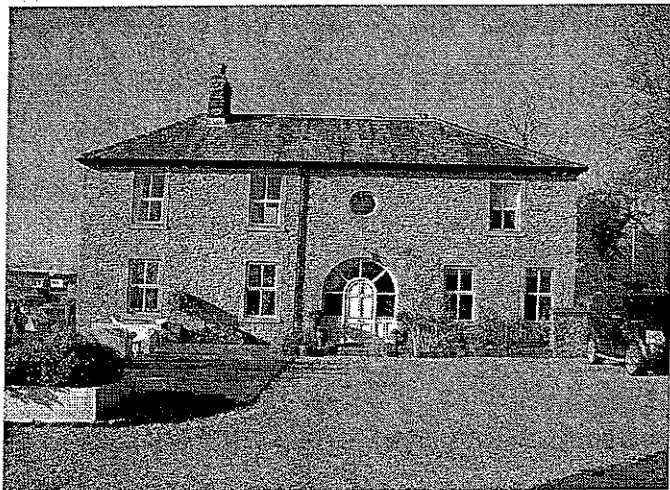
Fig 4. East elevation Gardeners Cottage
