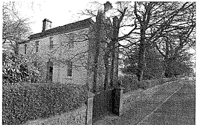
Fig 32 Dilworth House West elevation
