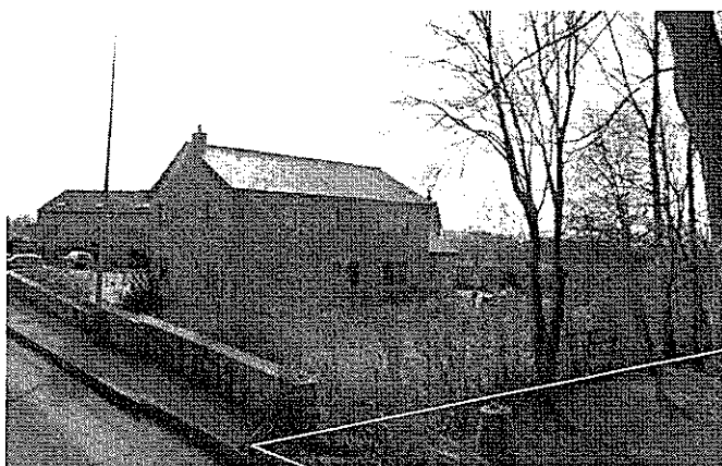
Fig 23 Dilworth Court residential development.
