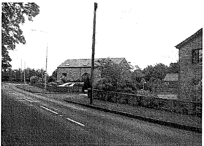
Fig 7 Dilworth Court residential properties
