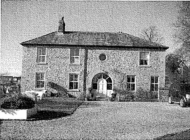
Fig 4. East elevation Gardeners Cottage
