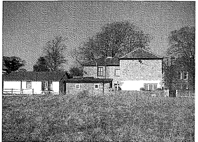
Fig 5 South elevation 39 (left) & 41 Dilworth Lane
