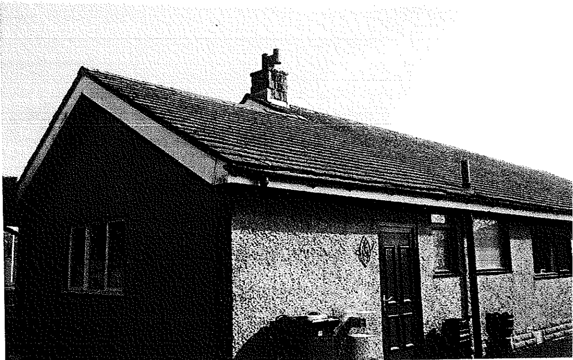
Photograph 4 - North corner of Garage
