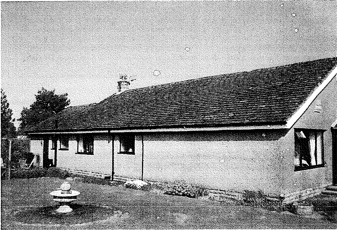
Photograph 3 - West (Rear) Elevation
