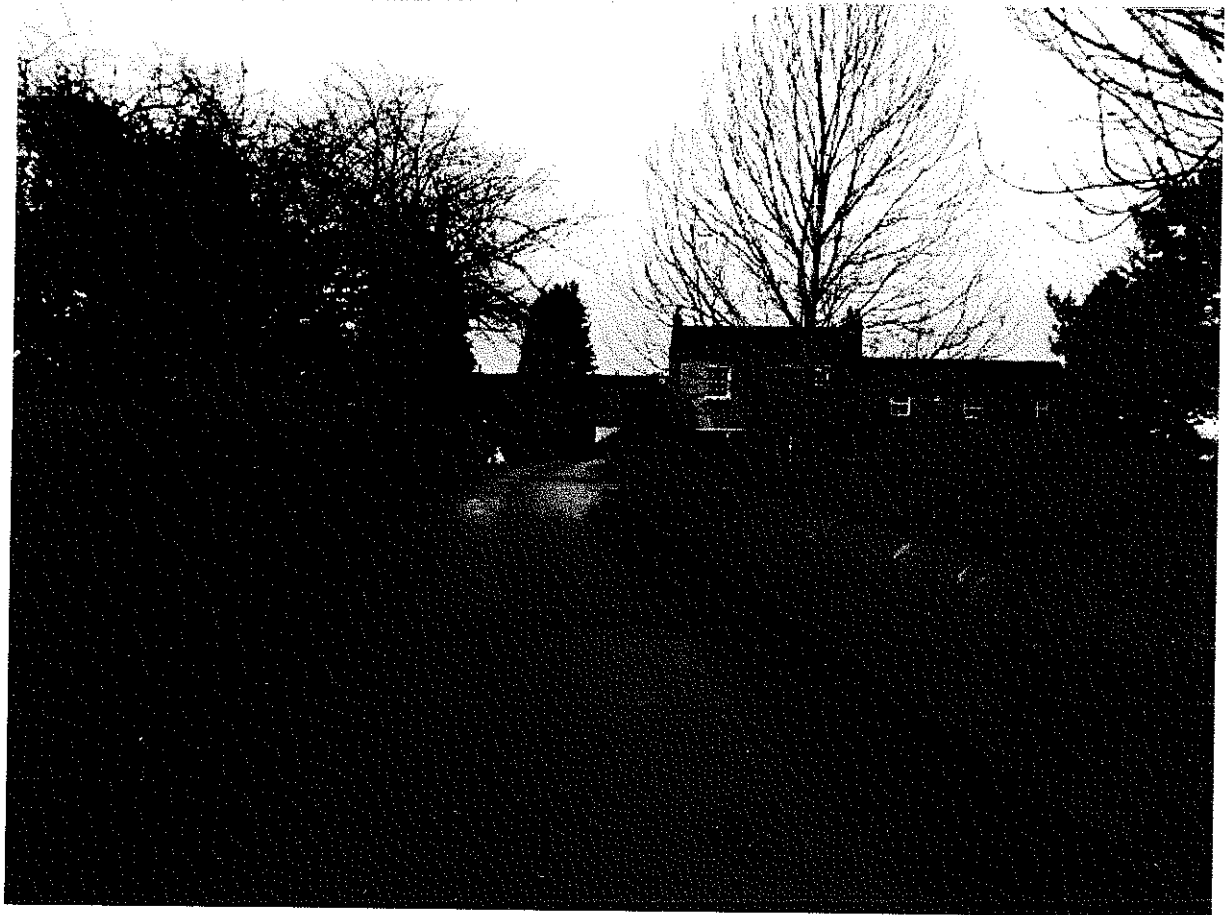
Photograph P5 – View west towards the Lower Standen complex taken from along the access road onto.
