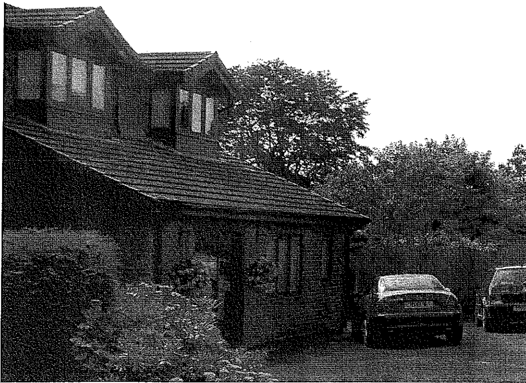
Dormer Windows at No. 4 Prospect Court
