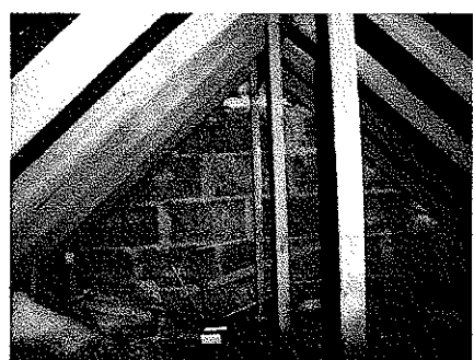
Figure 5: roof void at S gable end
