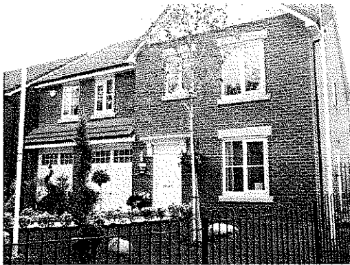
IMAGE OF COMPLETED HOUSE TYPE D1651(a) ON PLOT 1 (SHOW HOUSE)
