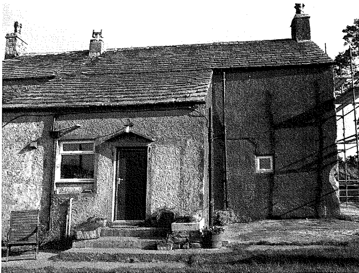
Figure 2: Photograph of existing rear elevation
