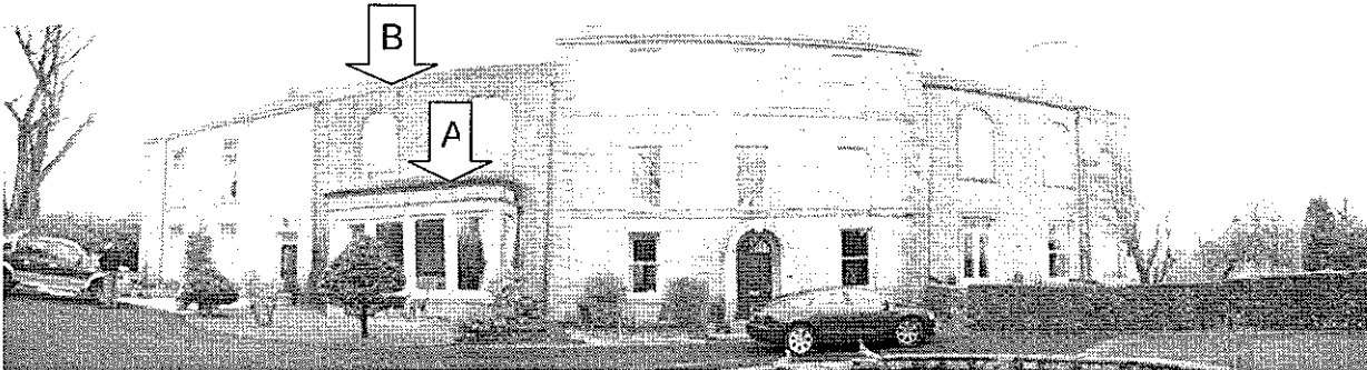
Figure 1: Front elevation No 5 Hodder Court is shown as area A the roof void shown as area 'B'
