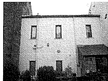
Figure 4: Rear view of property
