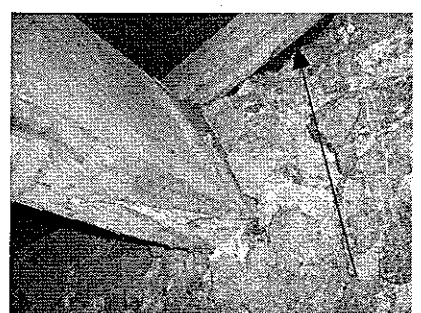
Figure 7: roof void B'
