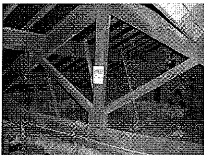
Figure 5: roof void B
