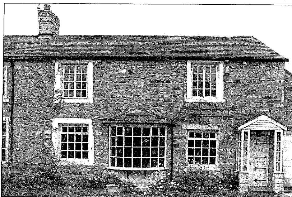
Photo 2: Front elevation of original cottages
