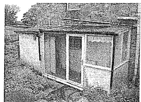
Figure 9: Lean-to at rear of property
