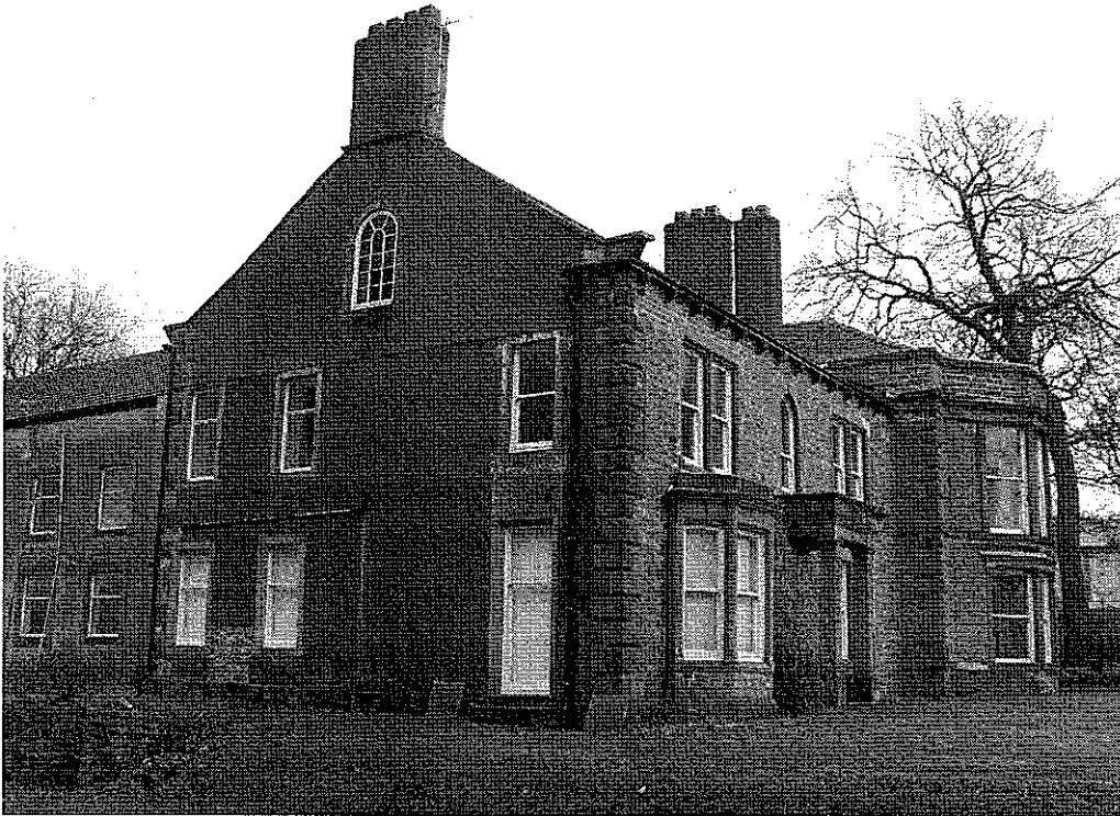
Fig 3: Photo of western gable elevation taken February 2009 after sample panel was exposed.
