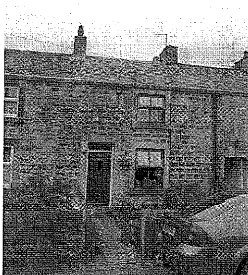
47 Avenue Road, Front Elevation
