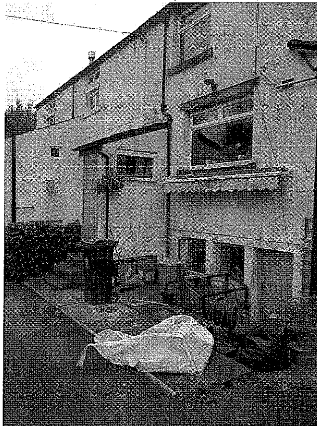
47 Avenue Road, Rear Addition
