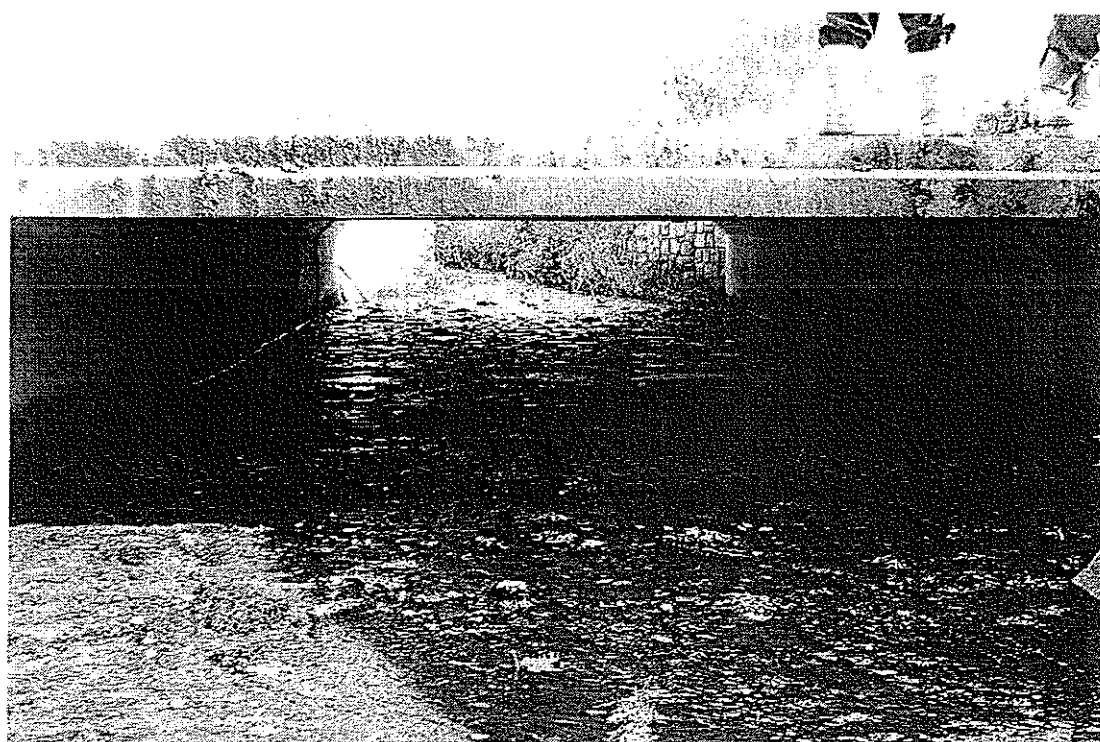
Culvert at Middle Lodge Road
