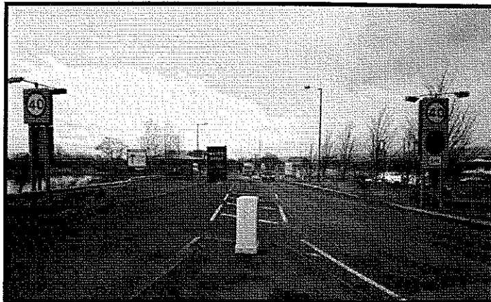
View along main access road from roundabout
