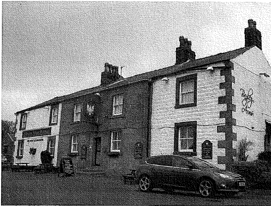
External Picture as Existing
