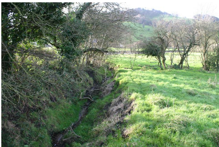
Plate 8- Open ditch with small flow open to field
