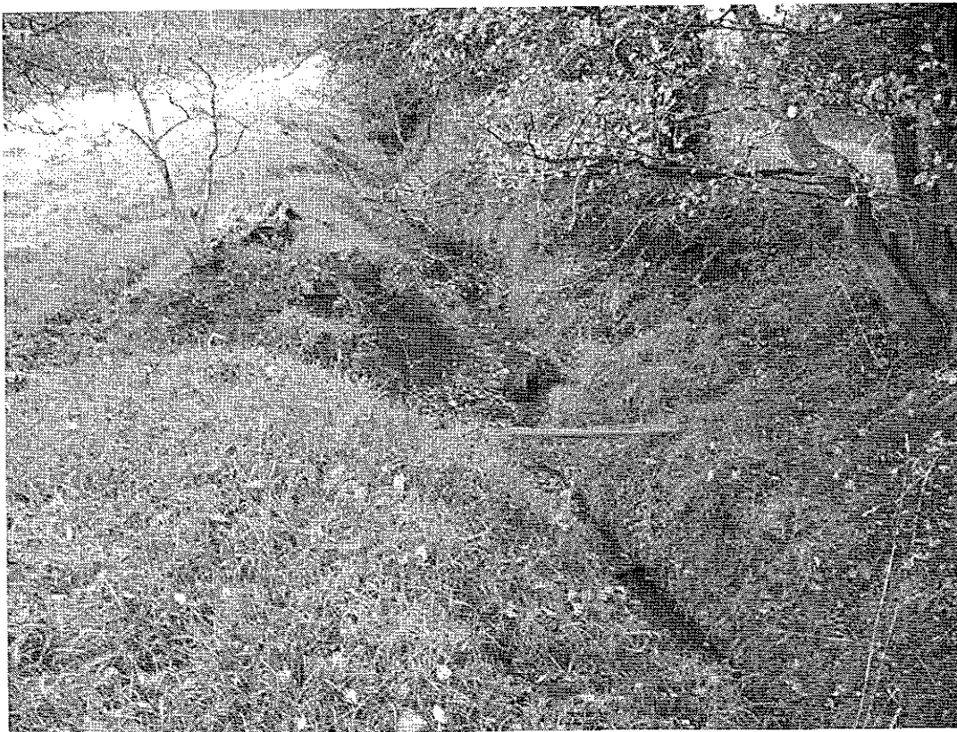
View to north of drain on eastern boundary
