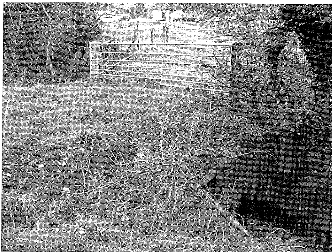
View to northeast of culverted section of drain and access path
